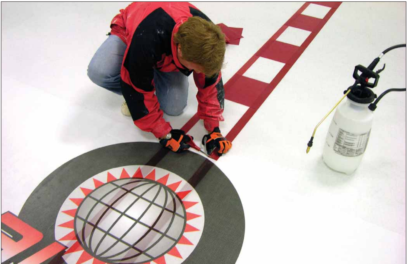
Vinyl mesh lines and logos offer the advantages of reusability and ease of application.
